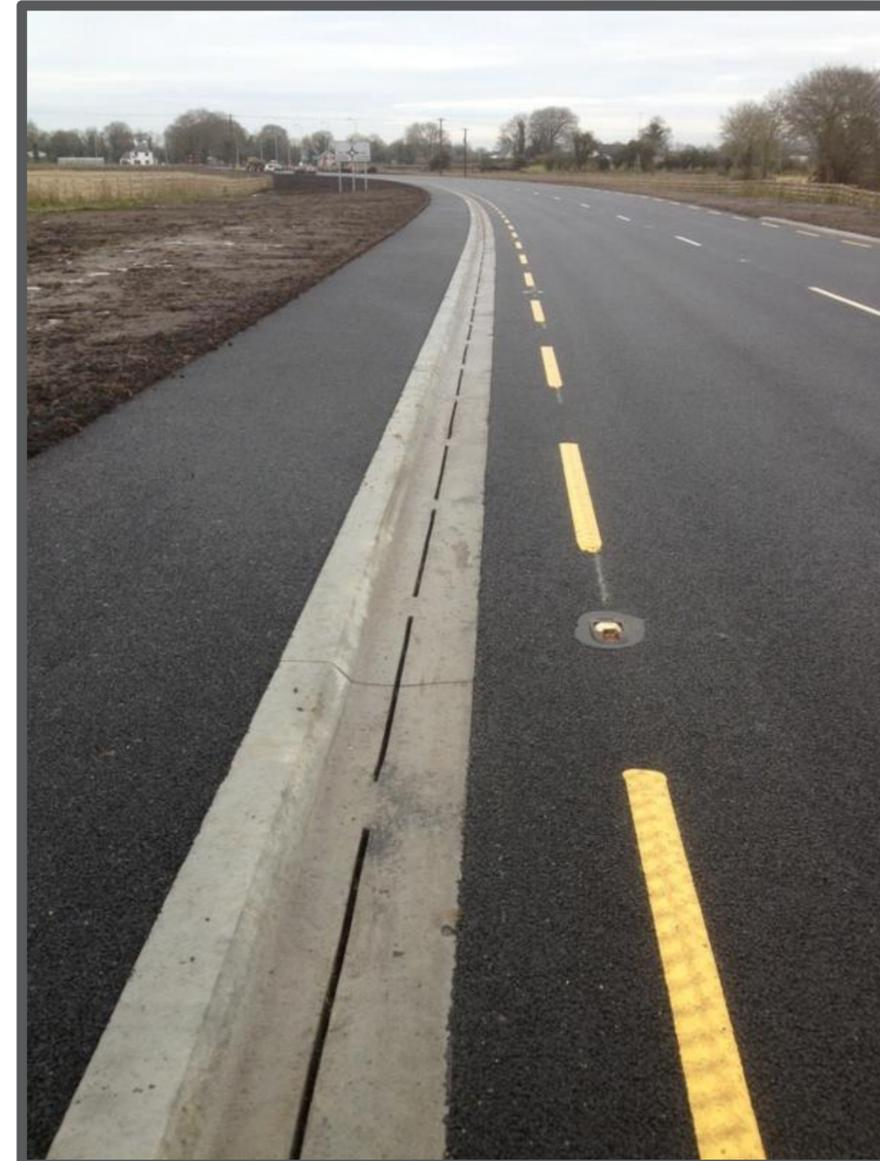
Near-side linear slot drains (no longer permitted under TII's standards).
