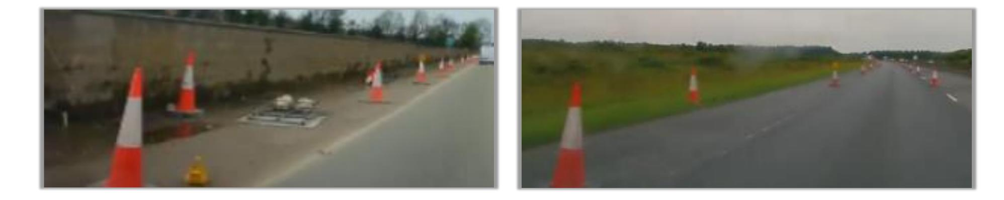
Cones were displaced and signs knocked over due to insufficient maintenance of TSM
