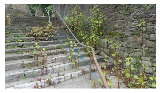
Figure 1 Japanese knotweed breaking through a paved surface [Photo: Arup]
