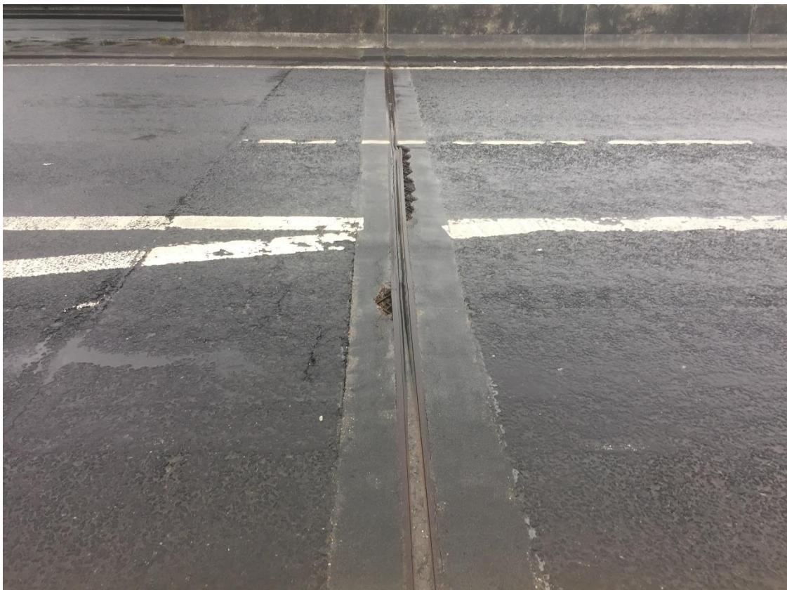
Photograph 8 Bunratty: Modular expansion joint with cracked nosing and delaminated nosing material around the helical reinforcement. The rail weld has failed. There is a crack between the nosing material and the pavement, and cracks in the pavement itself.
