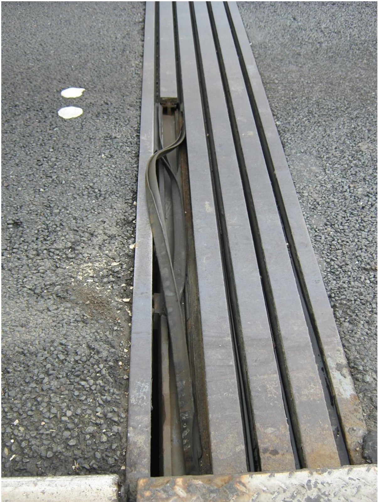
Figure D.2 Viaduct (precast prestressed concrete) built in 1993- The damaged rail has been taken out of the joint and corrosion is visible on the rails (Ref 1.I)
