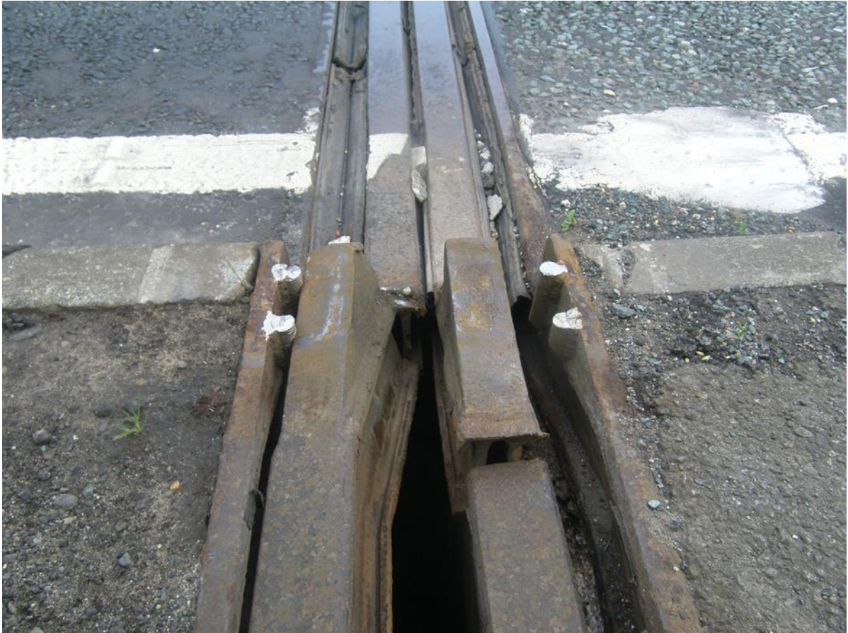
Photograph 4 Viaduct (Pre-cast pre-stressed concrete) Built 1976- Failure of joint footway. Seal failed between rails on carriageway (Source Ref 1.)
