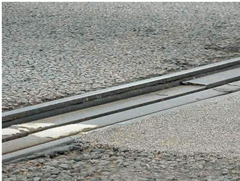
Photograph 6 Viaduct (in-situ concrete deck). Built 1986 - Damage to the west deck expansion joint - rail broken in the middle and level difference in carriageway surface. (Source Ref 1.I)
