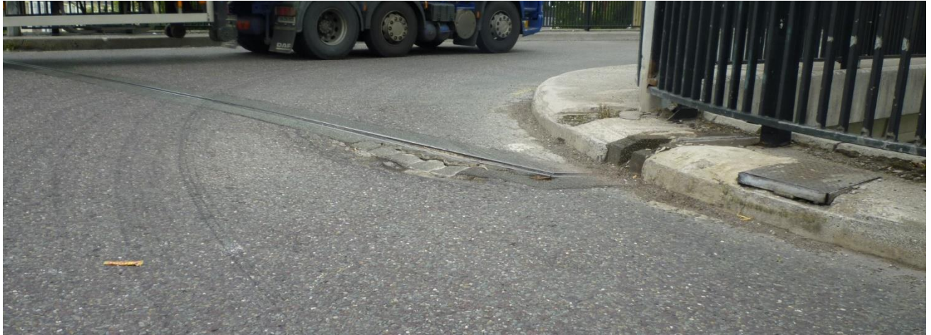
Photograph 9 Sliverspings; Modular expansion joint with failed nosing, exposed rail helical reinforcement and damaged surfacing adjacent to nosing. Failure due to excessive wear from heavy vehicles turning directly on the joint.
