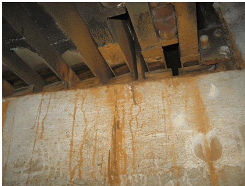
Photograph 3 Cable-stayed bridge (Composite steel-concrete deck) Built 1991 - Corrosion to expansion joint sliding plates over pier, circa 2007 (Source Ref 1.I)
