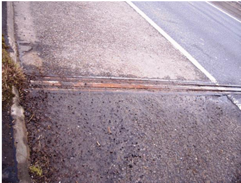
Photograph 7 Viaduct (in-situ pre-stressed concrete). Built 1990 - Corrosion to rails and debris in seals (Source Ref 1.I)
