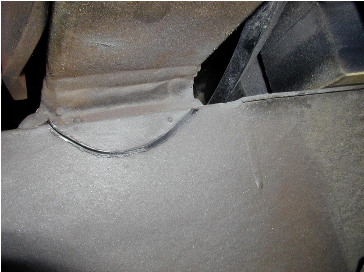
Photograph 1 Cable-stayed bridge (composite steel-concrete deck) Built 1991 - Fracture in the support joist immediately below the welded connection to the rail (Source Ref 1.I)
