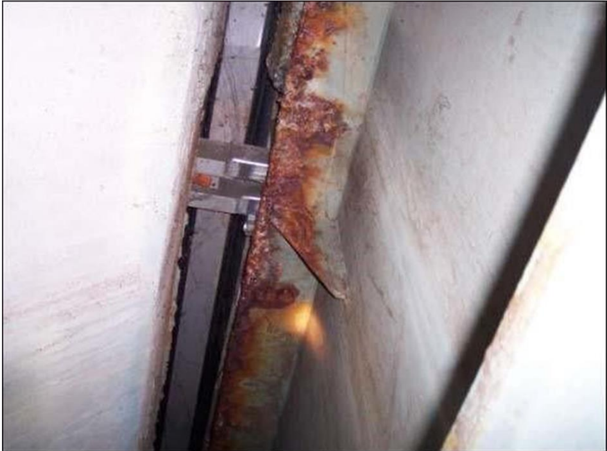
Photograph 5 Cable-stayed Bridge (composite steel-concrete deck). Built 1991 - Trimmer beam support steelwork corroded. (Source Ref 1.I)
