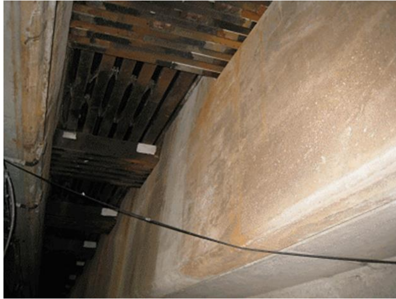
Photograph 2 Cable-stayed bridge (composite steel-concrete deck) Built 1991 - Rust staining from expansion joint over pier (Seal replacement stopped water ingress, circa 2007) (Source Ref 1.I)
