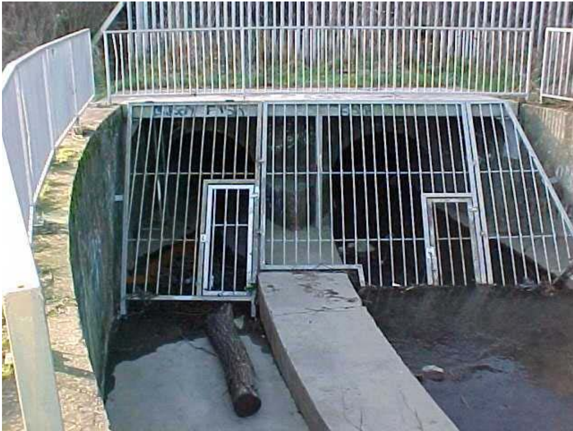
Plate A2: Example of a screen to a large watercourse
