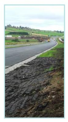
Combined filter drain on the N5 Ballaghdereen Bypass.
