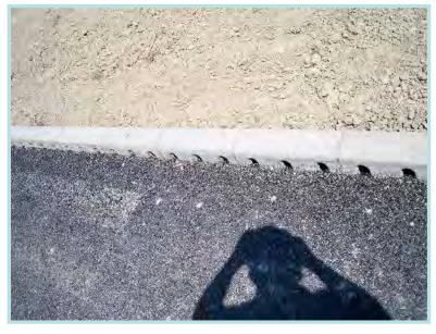
Example of combined kerb and drainage system on M3/N3 Clonee to Kells.
