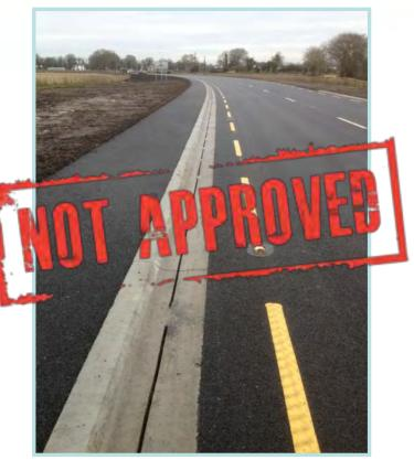
Nearside linear drainage channels.
