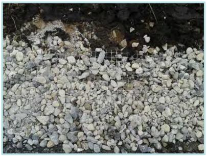
Surface of combined filter drain with geogrid.
