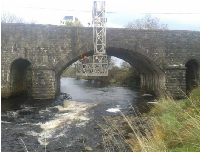
Coring to determine arch barrel depth
