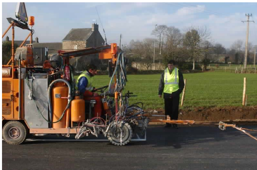
France: applying road marks
