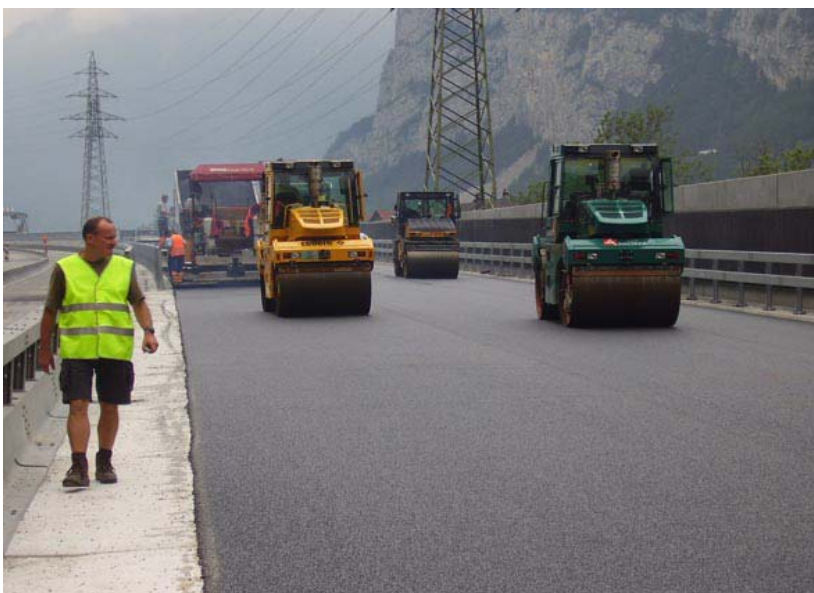
Switzerland: Paving on the St Gotthard
