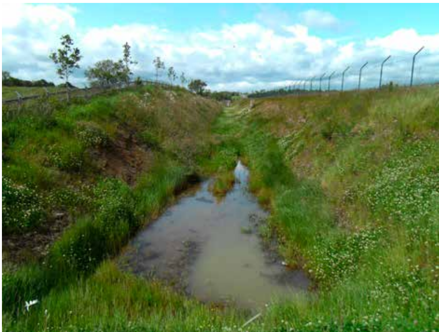
Plate 3 Linear attenuation ponds can become wetlands through naturally vegetation providing a permanent water table is present.
