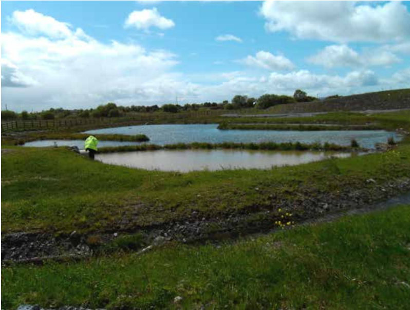
Plate 2 Wetland system with sediment forebay and berms.
