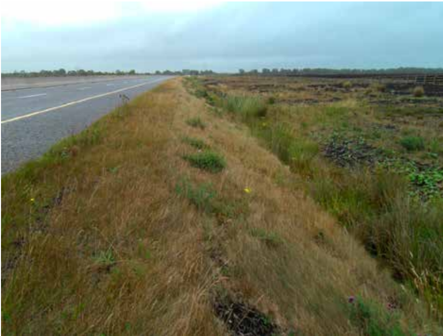
Plate 20 Linear wetland with wetland plants, constructed adjacent to the motorway, is used to convey and treat road runoff prior to discharging to either surface water or groundwater.
