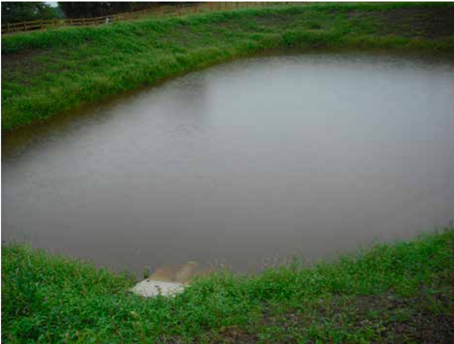
Plate 17 Simple detention basin with flow control structure.
