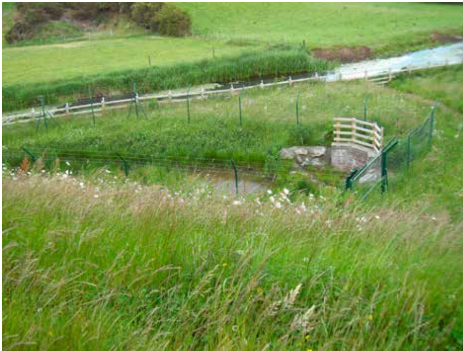
Plate 5 Small Detention basin adjacent to salmonid river. A detention basin will allow settlement of suspended solids prior to discharge. Control of discharge rates, through a suitable control structure, is essential to allow sufficient residence time.
