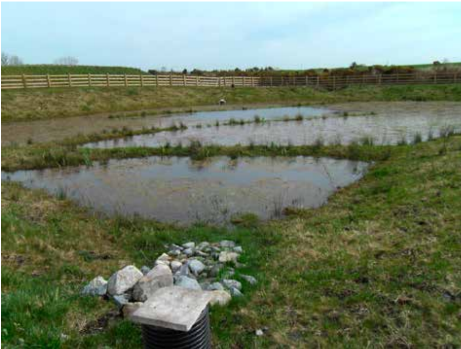
Plate 21 Hybrid Wetland with sediment forebay, berms and a range of water depths to promote different aquatic habitats.
