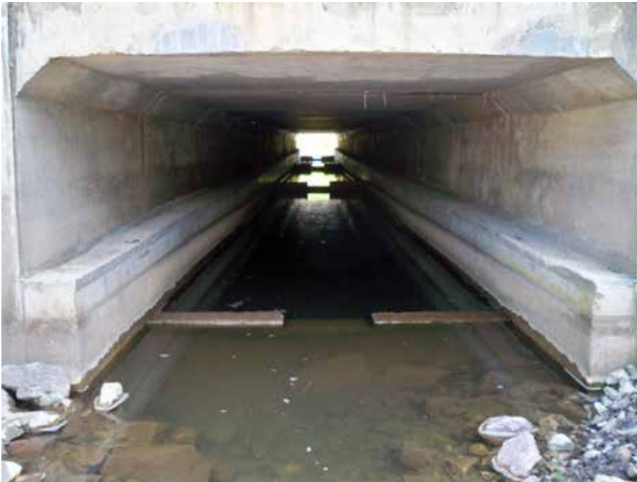
Plate 15 Box culvert with natural base to allow fish passage.
