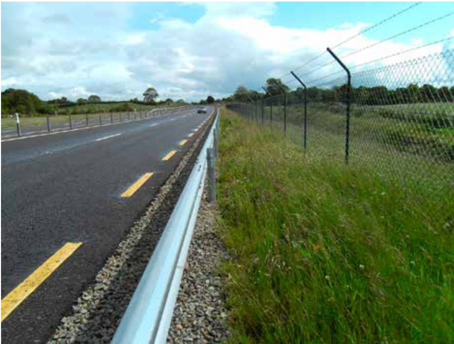
Plate 9 Filter Drain on low embankment. Newly constructed combined filter drain.
