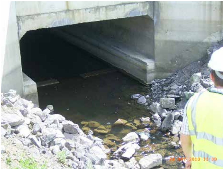
Plate 11 Box culvert with mammal ledge and flow control structures.
