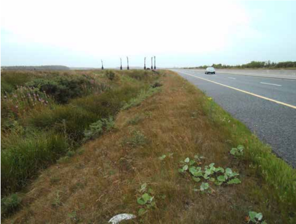
Plate 10 Linear wetland constructed adjacent to moteway. Runoff enters the linear wetland as sheet flow across a grass filter strip resulting in primary and secondary treatment prior to discharge.
